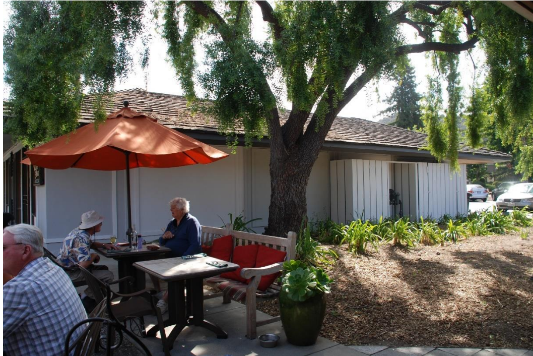
Figure 10. Building B, northwest façade, view southeast.
