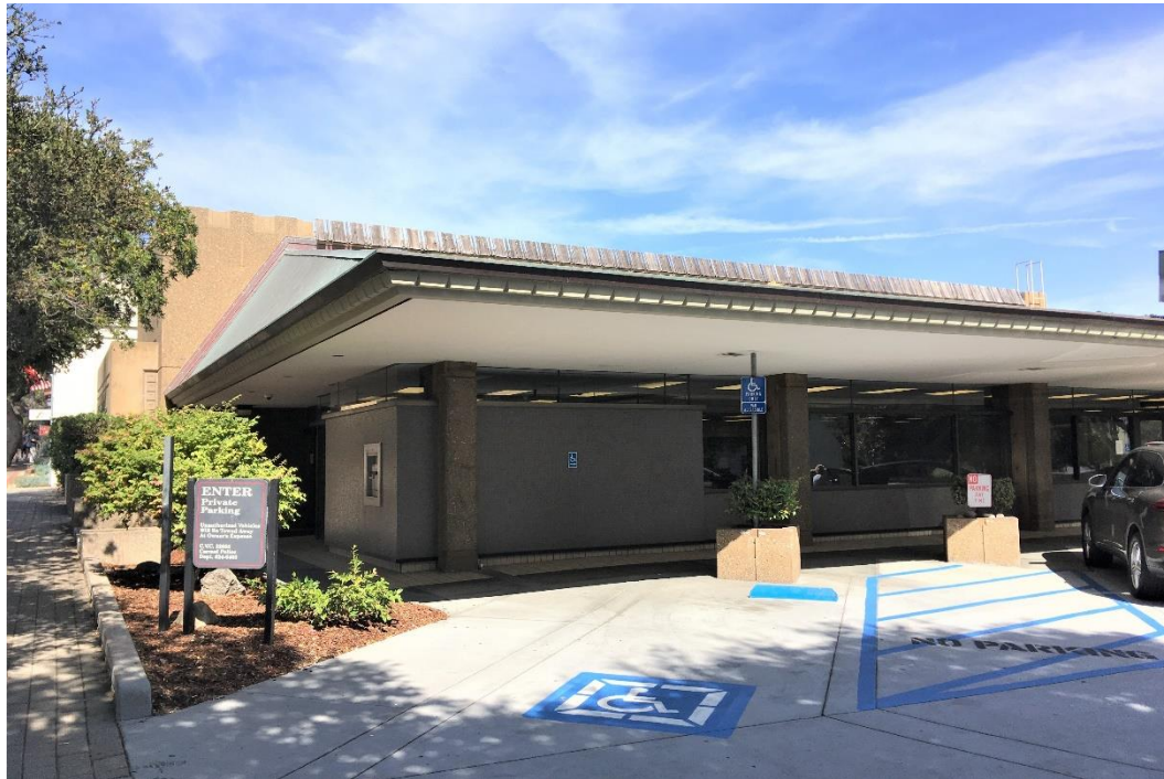
Figure 54. Wells Fargo building, Carmel-by-the-Sea, view northeast.
