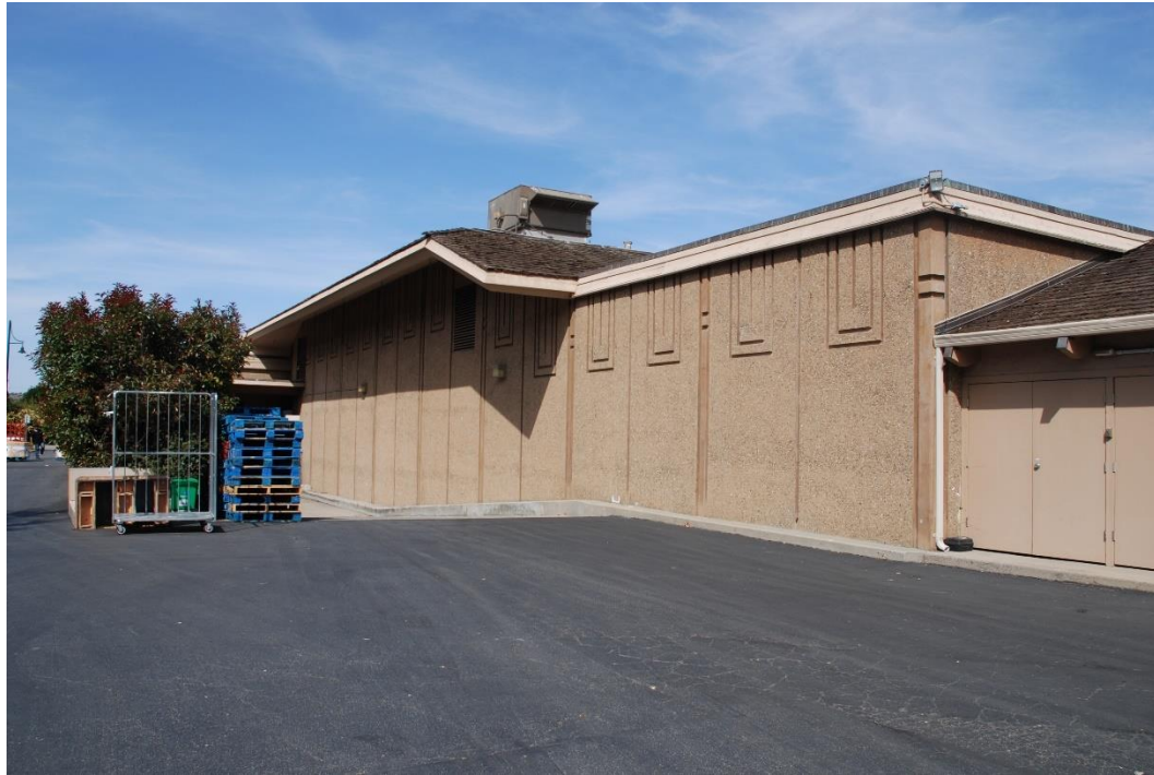
Figure 6. Building A, central portion of southwest façade, including Safeway loading dock, view northwest.
