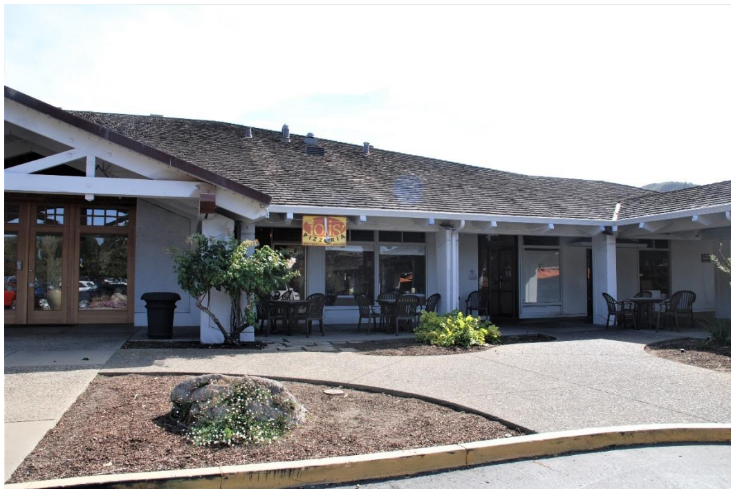
Figure 15. Building C, south portion of northwest façade, view southeast. Covered walkway attaches to Building C roof at right.
