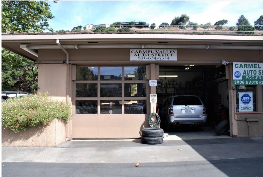
Figure 26. Building E, roll-up doors at west side of southwest façade, view northeast.
