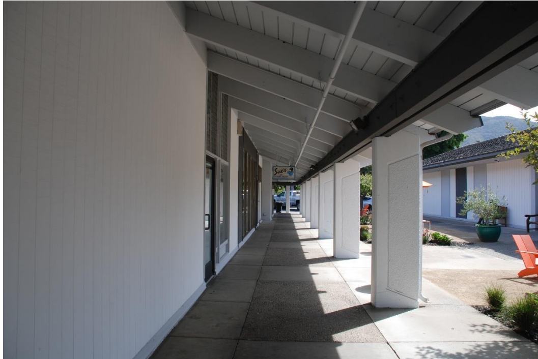
Figure 17. Building C southwest façade, view southeast.
