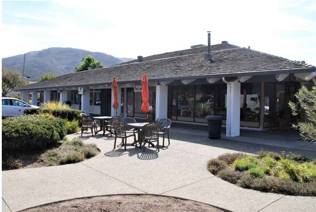
Figure 20. Building C, northeast façade, view southeast.
