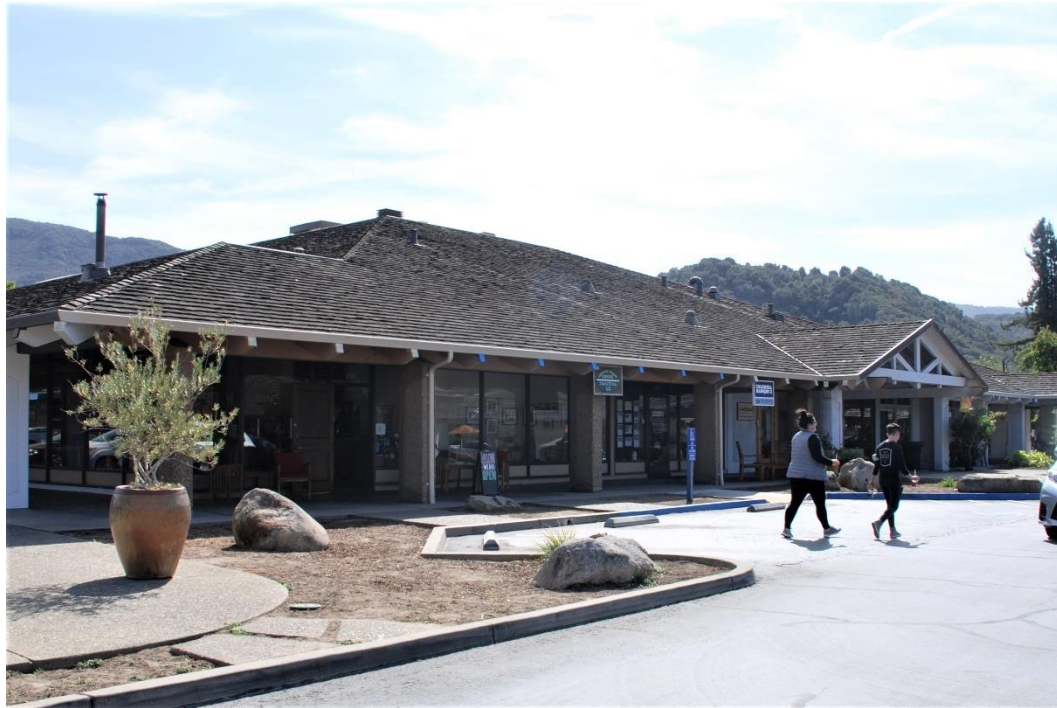
Figure 14. Building C, northwest façade, view south.
