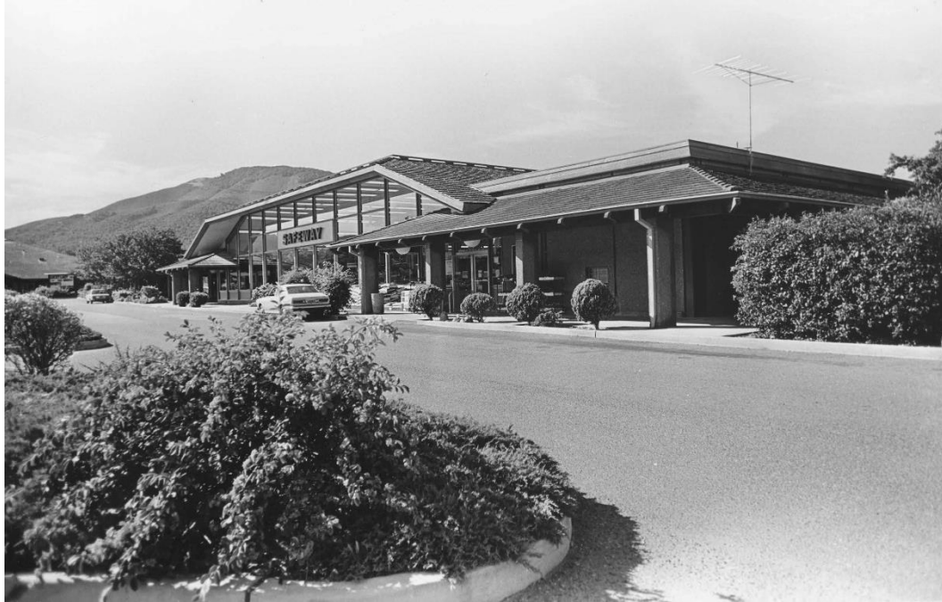
Figure 37. Building A, ca. 1974, view southeast.
