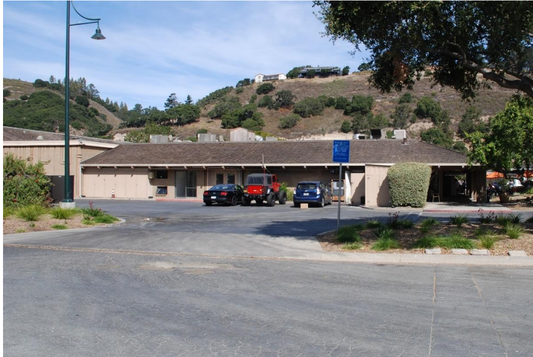
Figure 7. Building A, southeast portion of southwest façade, rear of stores to southeast of Safeway, view northeast.
