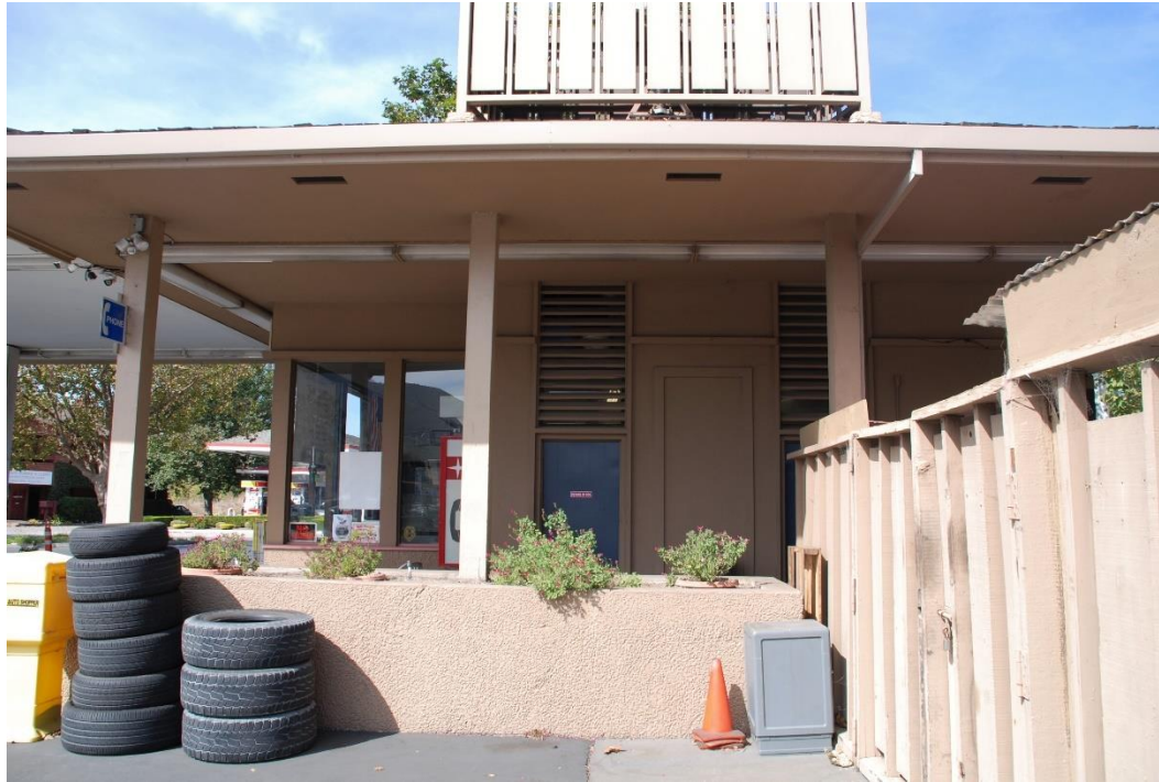
Figure 28. Building E, southeast façade, view northwest.
