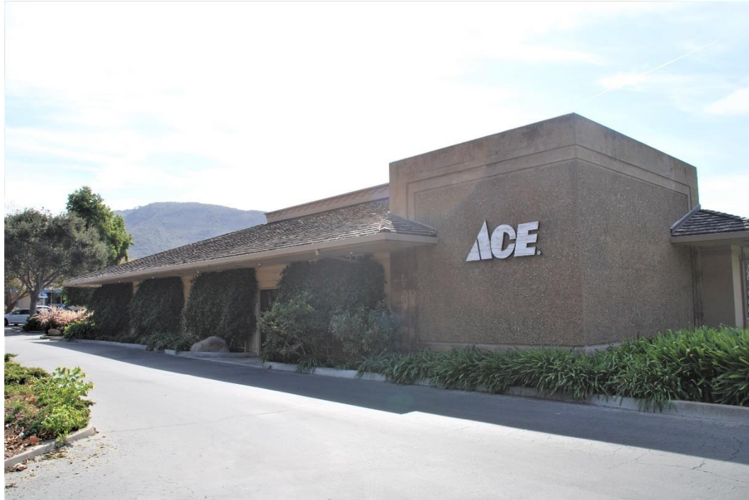
Figure 22. Building D, northeast façade, view southeast.
