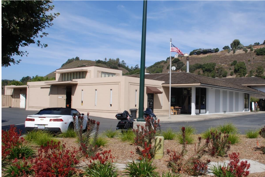
Figure 12. Building B, east portion of southwest façade and southeast façade, view north.
