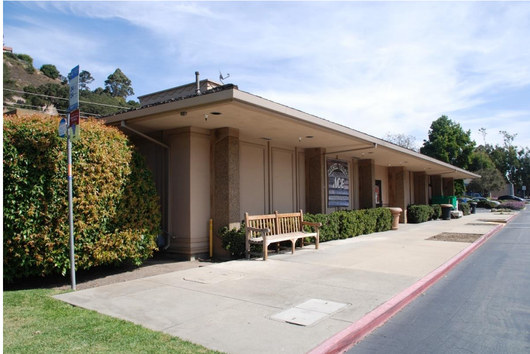
Figure 24. Building D, southwest façade, view east.
