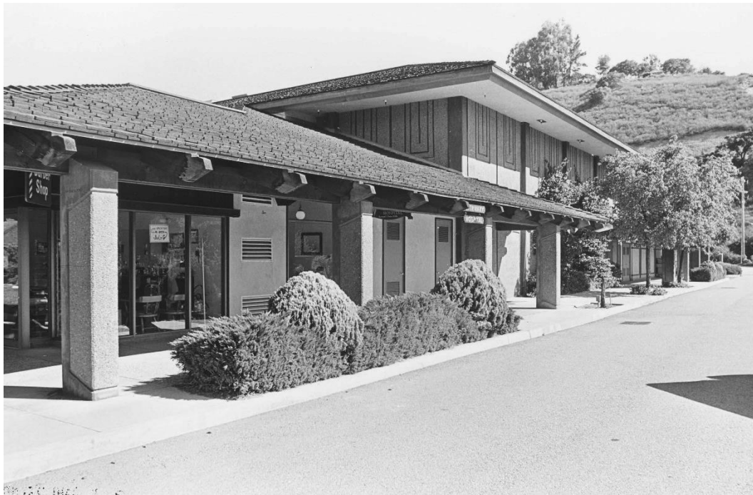
Figure 38. Building C, ca. 1974, view north.
