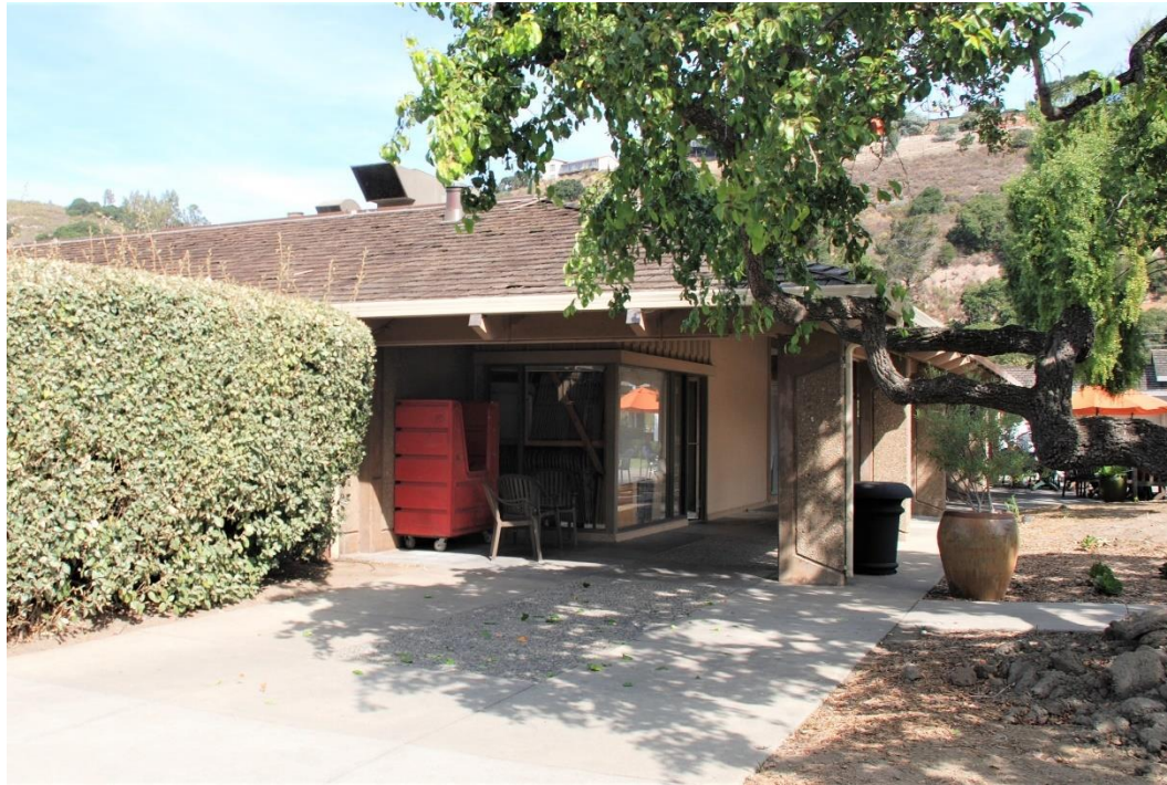
Figure 8. Building A, view northeast across southeast façade.
