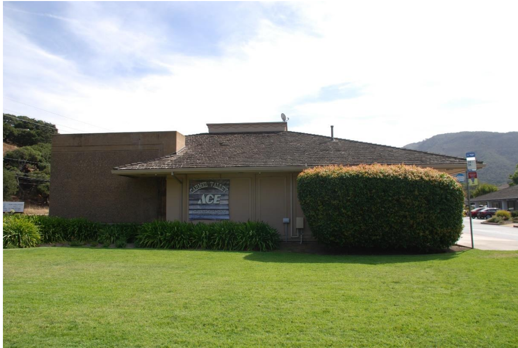
Figure 23. Building D, northwest façade, view southeast.
